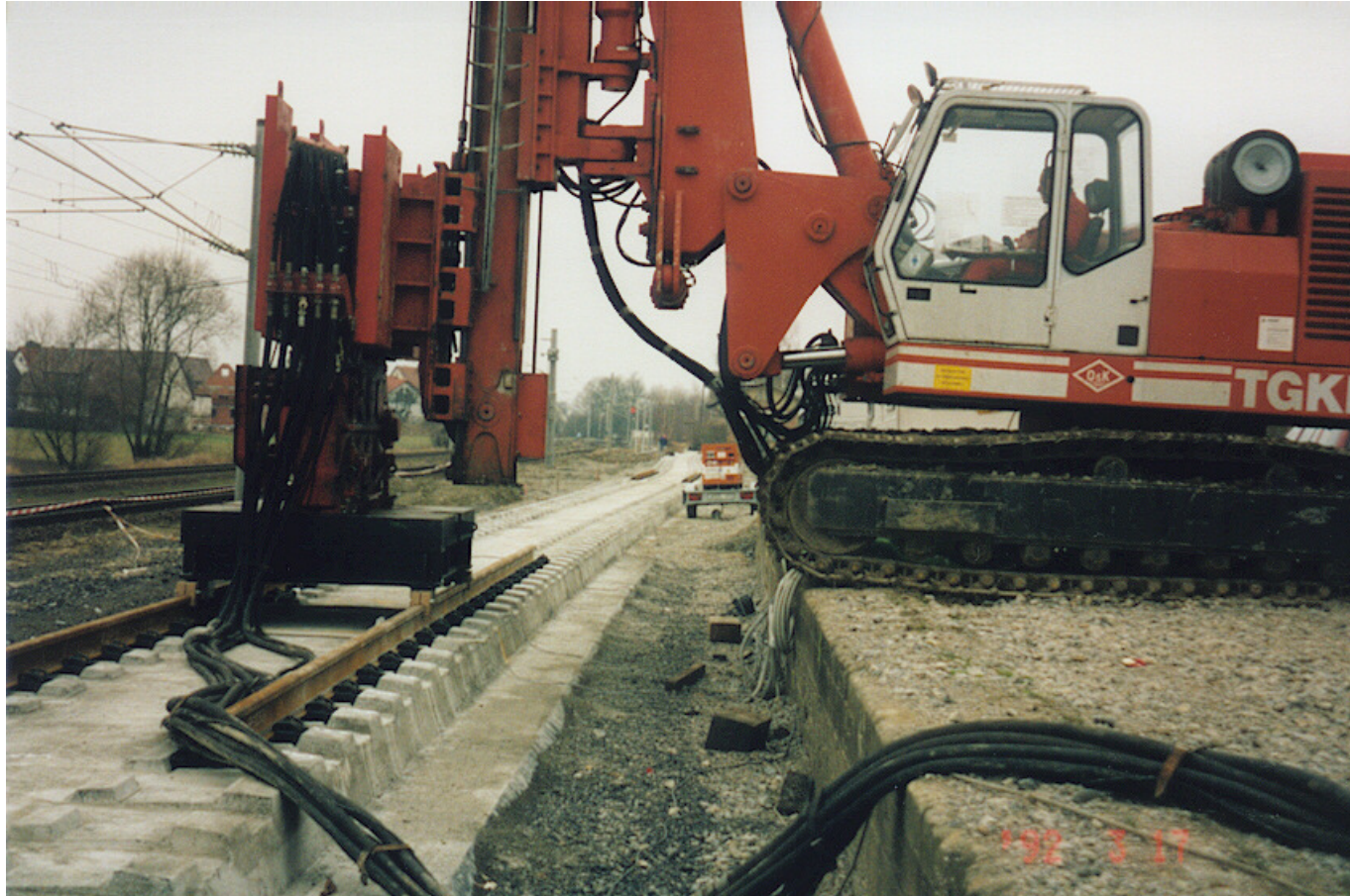
Field test with slab track in Eckartshausen
